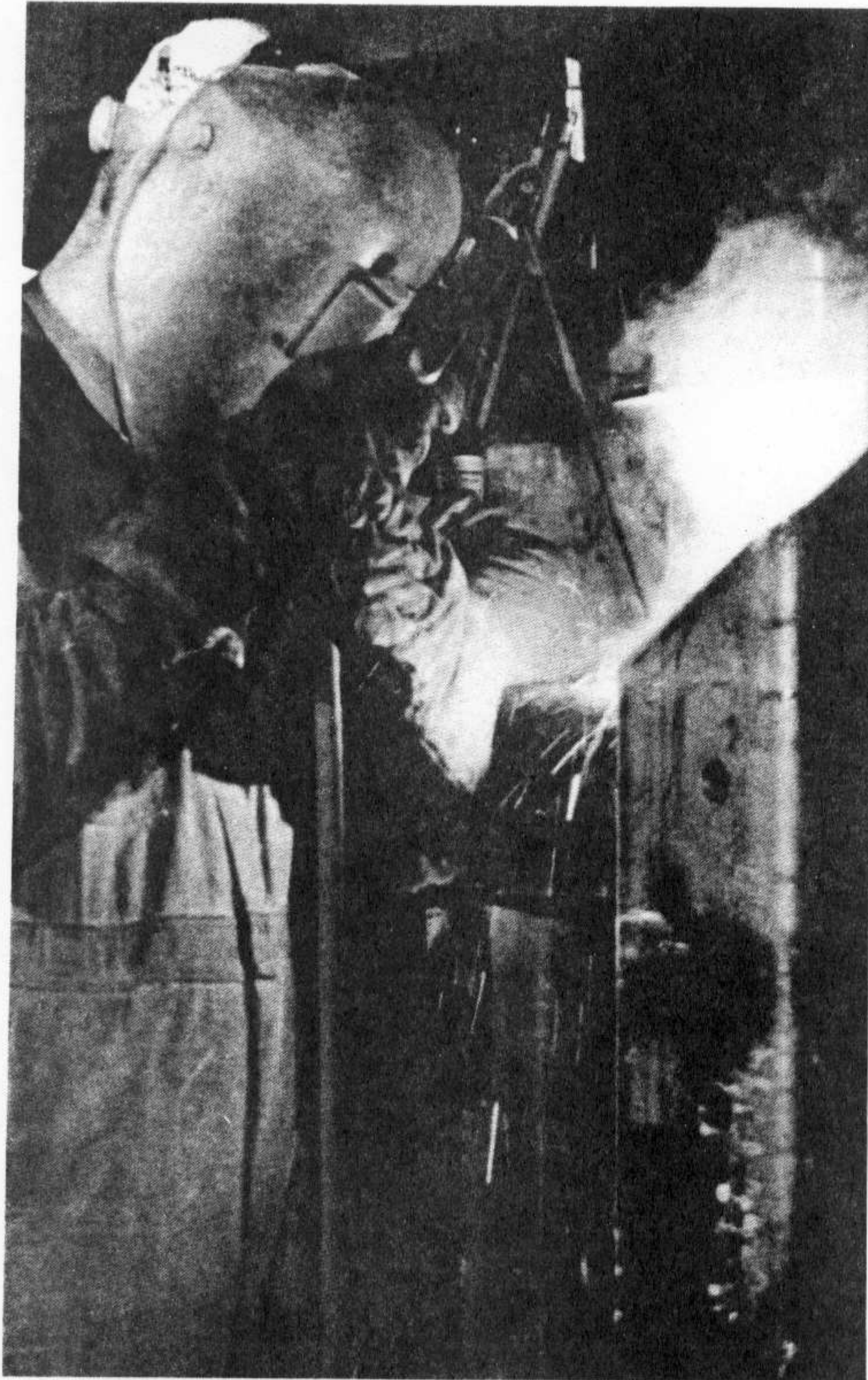
Large weldment, built up by automatic submerged arc and semiautomatic welding, is given finishing touches by manual stick-electrode welding.
